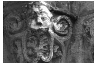
Nouvion tower level 1 1103
