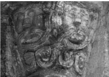
Nouvion tower level 1 1103
